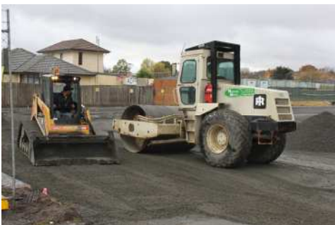
Michael White and his team work on Sports Centre Car Park
