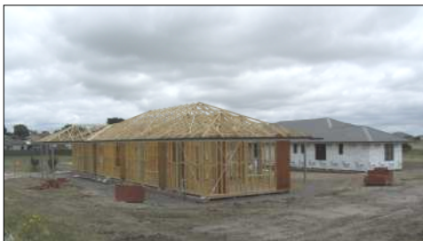
Medical student accommodation under construction in Quinn Crescent, Kyneton
