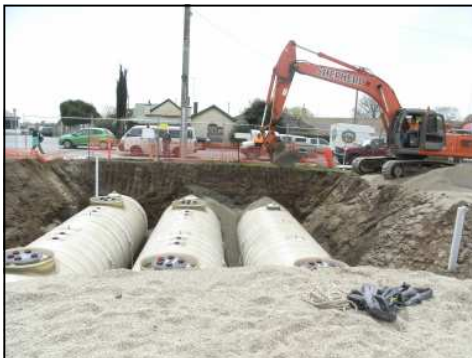
The underground tanks for the new Servo
